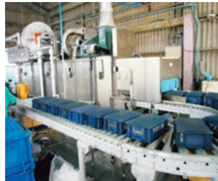
Plastic container washing line
