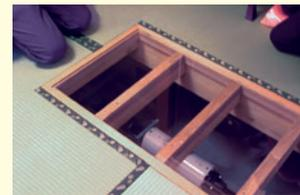
Seismic isolation devices installed in their own house. One tatami mat has been replaced with glass, enabling clients to view the installation.
