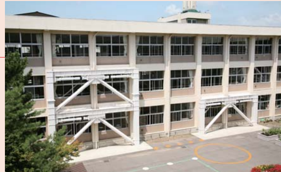
Exterior of the Chikuzan elementary school building in the city of Akita after the installation of viscous dampers for quake-resistance
