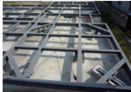
Foundation for a residence, built by Haneda Construction.
