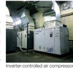
installed at the KOFU Plant
