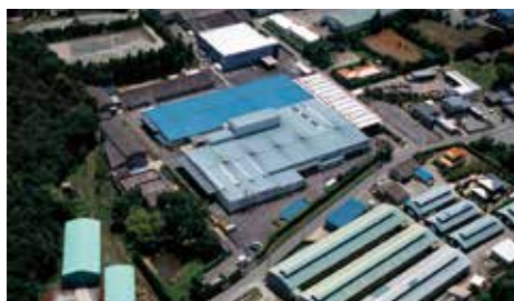
● Mie Plant 三重工場 Site: 42,259 m 2 (454,872 sq. ft.) / Floor space: 25,405 m 2 (273,457 sq. ft.)
