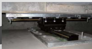
Seismic Isolation System
