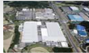
Yamaguchi Plant Renewal
