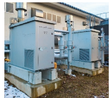
Hot water boiler
