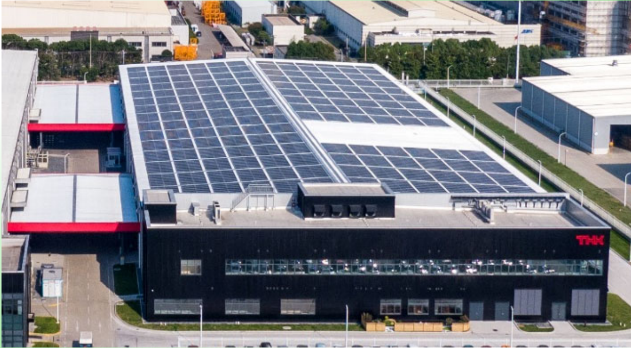
Solar Power Generation (THK Changzhou Plant)
