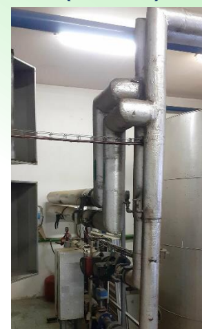
Compressor exhaust heat being utilized (TRA Czech)
