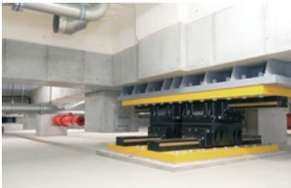
Seismic Isolation System Linear Re-circulating Guide Model CLB
