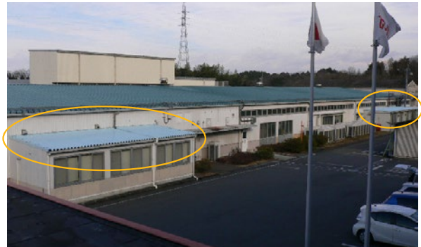
Quality Assurance Section office (left) and Manufacturing Section II production floor office (right) with coated roofs
