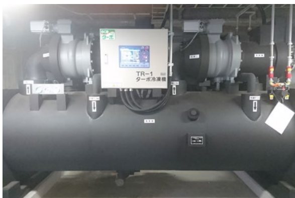
New inverter-type turbo chiller
