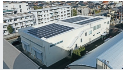
Mishima Plant THK INTECHS CO., LTD. Solar power generation
