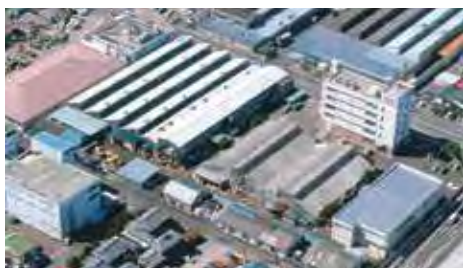
●THK INTECHS CO., LTD., Mishima Plant Site: 12,917 m 2 (139,038 sq. ft.) / Floor space: 10,447 m 2 (112,451 sq. ft.)
