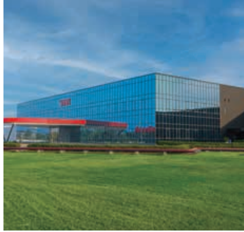
● THK India Pvt. Ltd. India Headquarters and Sri City Plant
