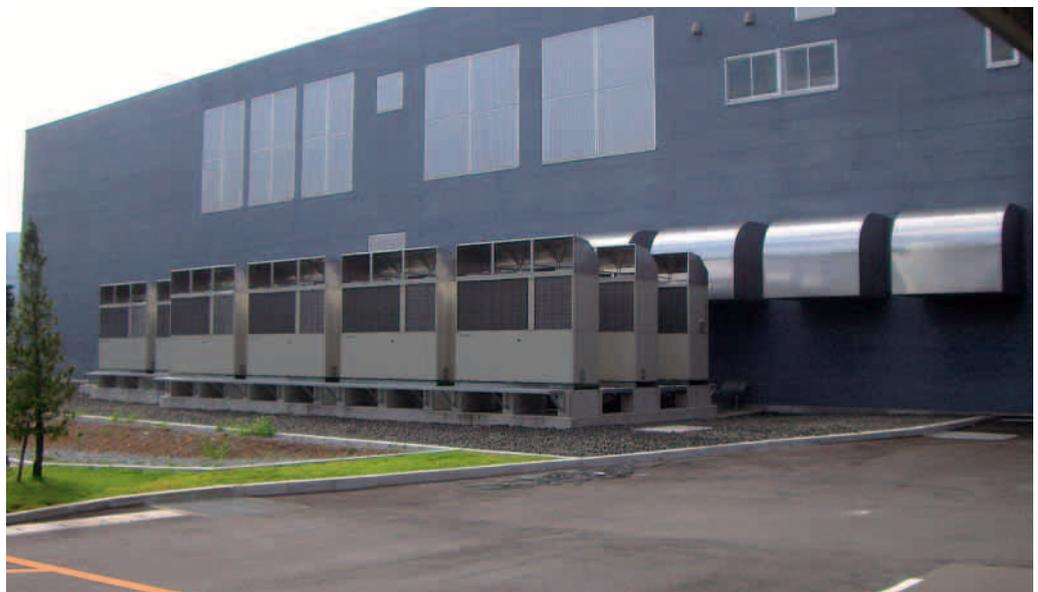
Gas-fired heat pumps that run on LNG (Chubu Distribution Center)
