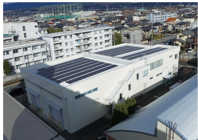
Solar panels installed on top of the development building
