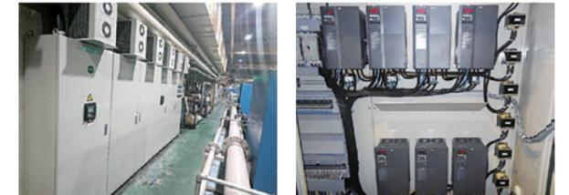
Inverter control panels added to Factory 3's centralized coolant system
