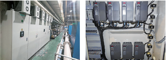
Inverter control panels added to Factory 3's centralized coolant system
