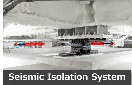
Seismic Isolation System
