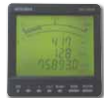
Power consumption at THK NIIGATA was monitored over a six-month period.
