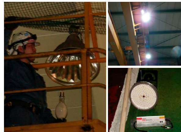
(Left) Removing mercury bulbs at the Sendai plant (Top right) Lighting after the LED upgrade (Bottom right) Newly installed LED light
